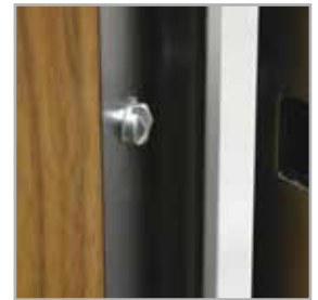
levering protection bolts
