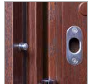
levering protection bolts
