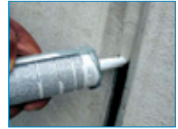
Backerseal behind field-applied liquid sealant provides true "belts and suspenders" sealing – 2 systems working on different principles to guarantee performance of the same function.
