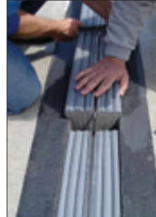
The back pressure of the SJS foam and an epoxy adhesive provides watertightness with non-invasive anchoring without relying on a gutter. Installation is faster than other more complicated systems.
