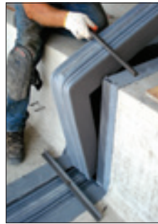
EMSEAL offers pre-fabricated factory transitions for treads and risers which allow for ease of installation and which also ensure watertightness in changes of plane.
