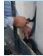
Backerseal behind field-applied liquid sealant provides true "belts and suspenders" sealing – 2 systems working on different principles to guarantee performance of the same function.
