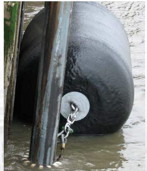
Foam filled floating fender with steel construction, following the tide up and down
