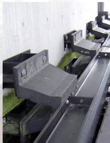
Fenderguiding with archfenders and steel construction with sliding bars of HD-PE
