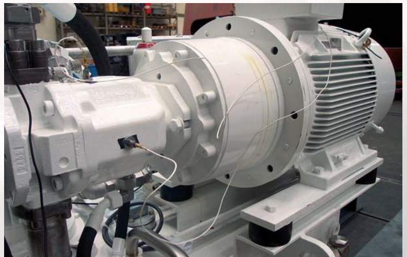
Vibration measurements on site
