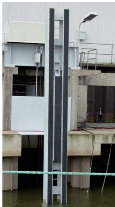
Fendersystem with rubber fender and sliding bars
