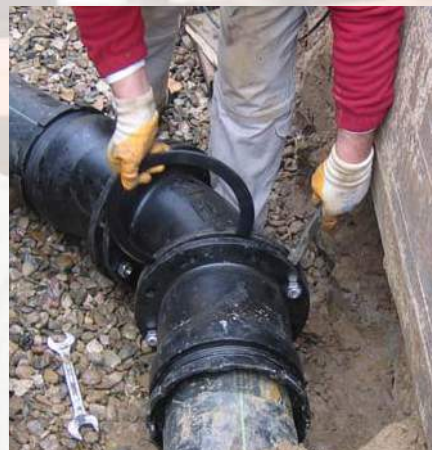
Wedge-shaped gasket for underground conduits
