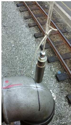
The 'missing' photograph showing the centre pop and plum bob.
