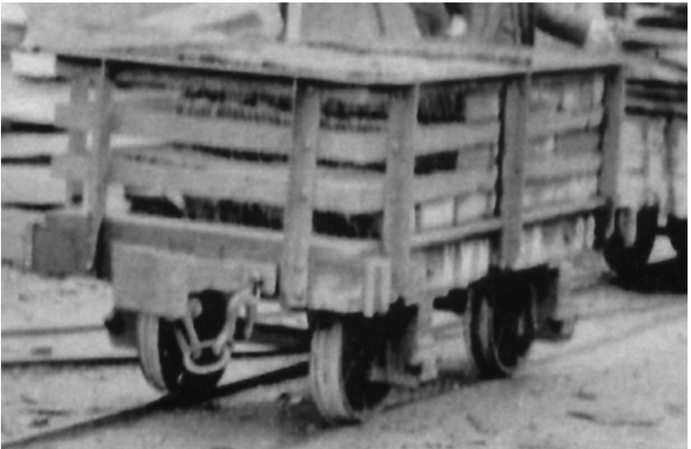
Photo 7 - NWNGR slate wagon no. 88 at the mills below Hafod y Wern Quarry, Bettws Garmon. The photograph was taken at some time between the summer of 1890 and March 1898 - Dafydd Walter Dafis collection/Gwynfor Pierce Jones.
