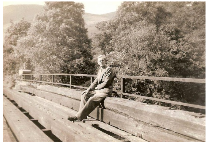
Michael Davies at the Afon Treweunydd (Glanrafon) 'Viaduct' - 18 th June 1954
