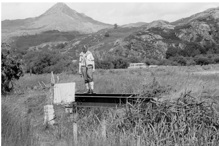
The walk that included the previous 3 photos ended at Croesor Junction. Described by David as John's favourite photo, here we see John Keylock standing on the girders that carried the WHR over a small ditch. The photo was taken some years before the survey walks. Arch 4462
