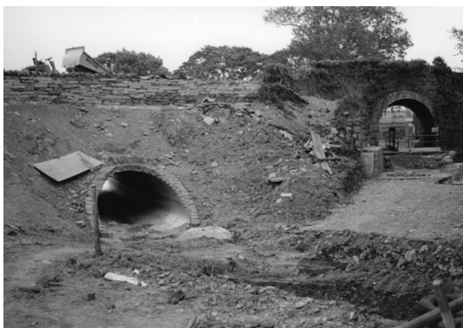
Rebuilding at Cae Moel, looking towards Tryfan Junction.
