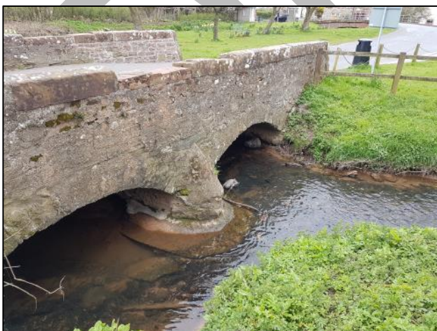
Photograph 9: Warcop Bridge over the Lowgill Beck
