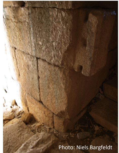
Fig. 7: A junction where the interior corridor can be sealed off.
