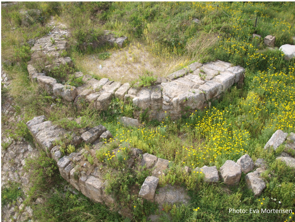
Fig. 1: The northernmost Hellenistic tower. Today it can be seen from Waygand street, where it is bridged over George Haddad street.
