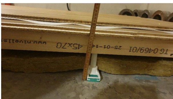
Figur B4.8: Montering prov M15.
