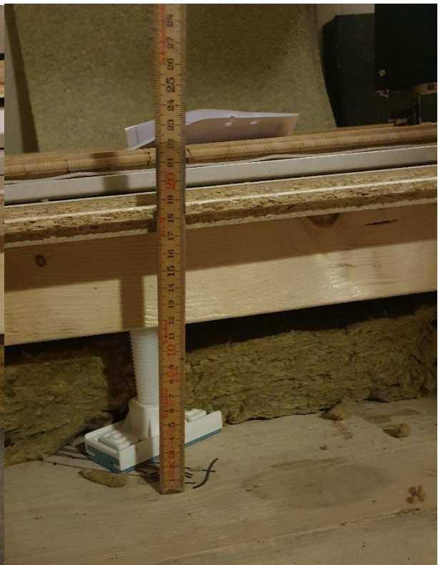
Figur B4.16: Montering prov M13.
