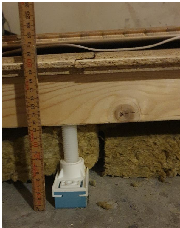
Figur B4.17: Montering prov M5.
