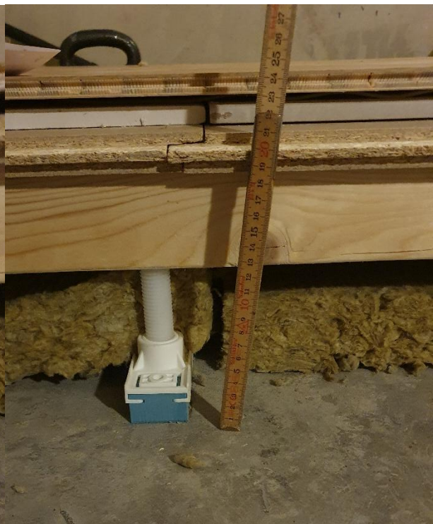
Figur B4.20: Montering prov M6.
