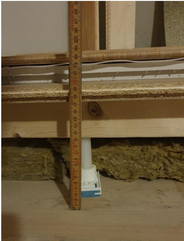
Figur B4.15: Montering prov M14.
