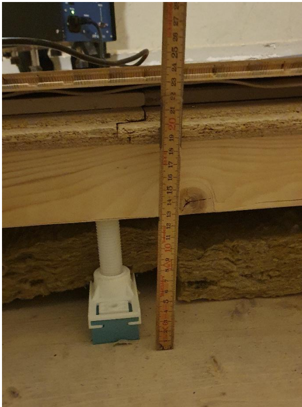
Figur B4.11: Montering prov M2.
