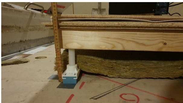
Figur B4.5: Montering prov M1.
