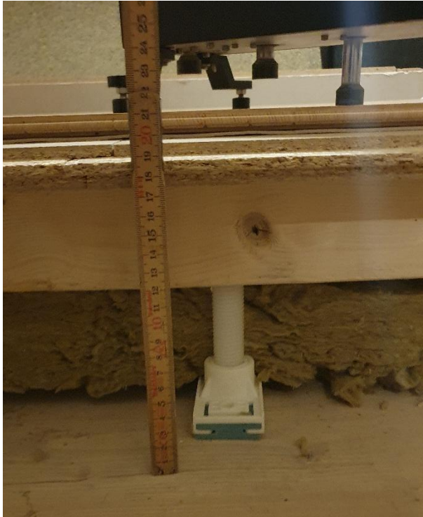
Figur B4.18: Montering prov M12.
