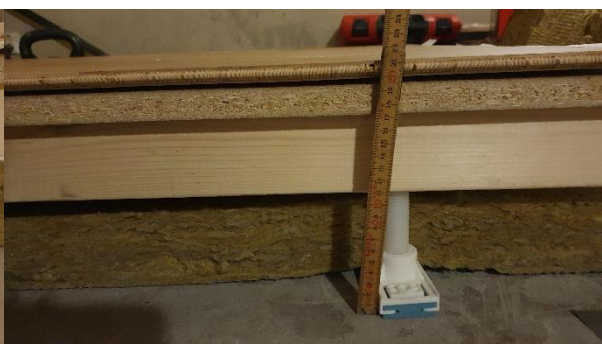
Figur B4.7: Montering prov M9.
