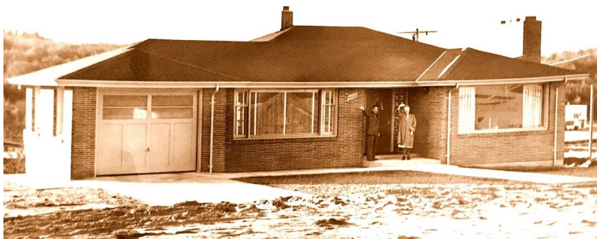
Picture of Lena Woien and Conrad Westerberg at their new home in Everett, Washington in 1950. Conrad built the house.
