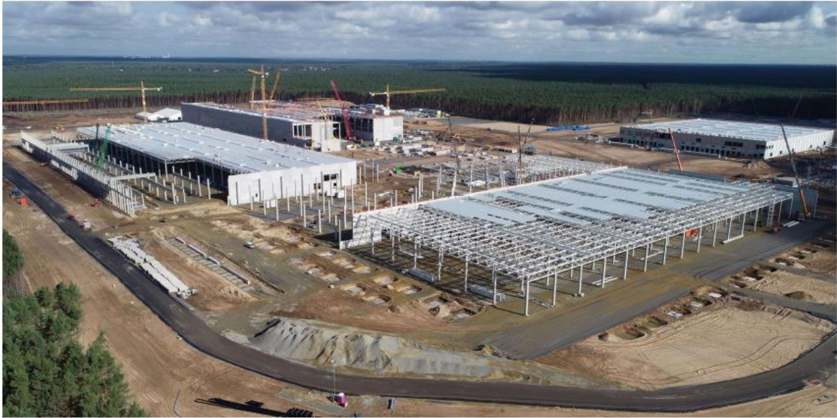
GIGAFACTORY BERLIN - MODEL Y FACTORY CONSTRUCTION
