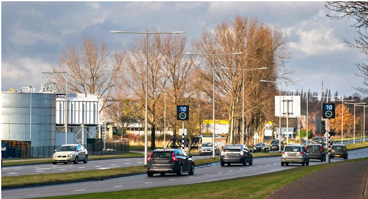
Figure 18: Speed advisory sign to achieve green wave on arterial road (Source: Dick Vermaas)
