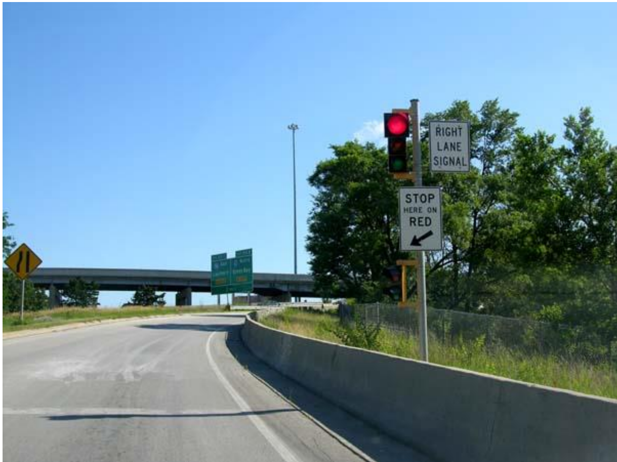
Figure 14: Ramp metering in the US 1 .
