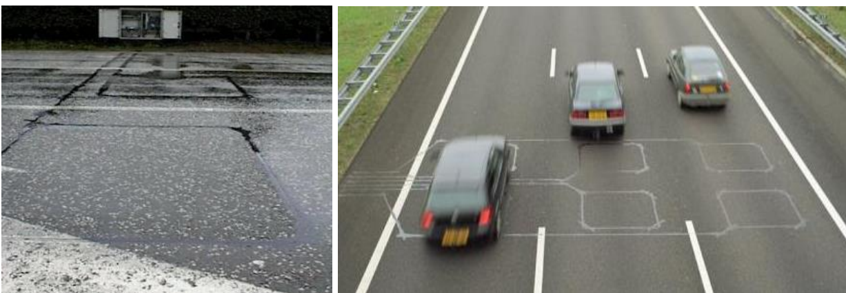
Figure 28 Inductive loop detectors on the urban road (left) and motorway (right). (Source: Henk Taale, ITSEDULAB)
