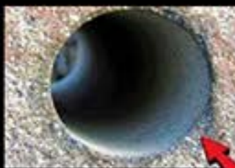
Core drill hole in concrete by modern power tools
