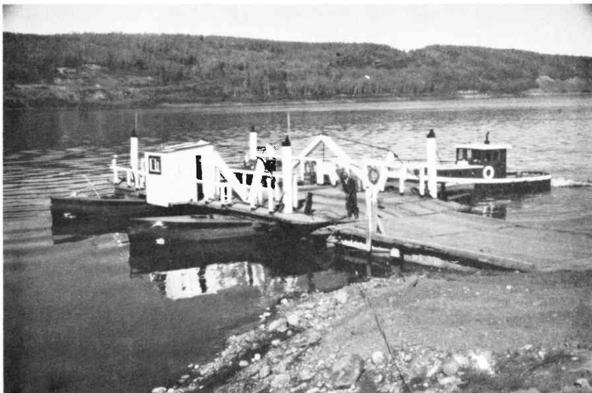
FIGURE 8 - The existing La Crete ferry
