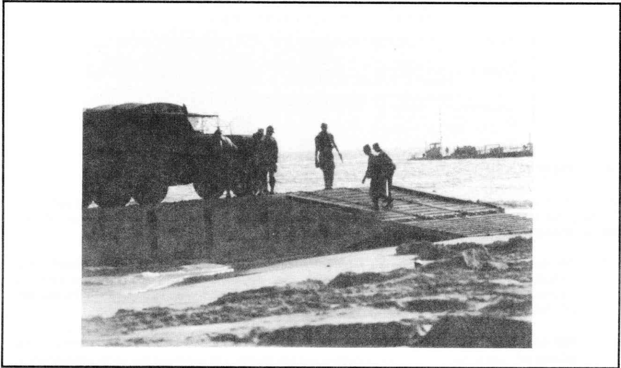
Figure 1. Causeway Ferry Offload On Steep Beach
