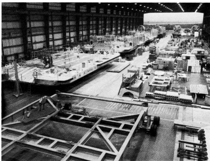
Figure 7: Production Line at TMS
