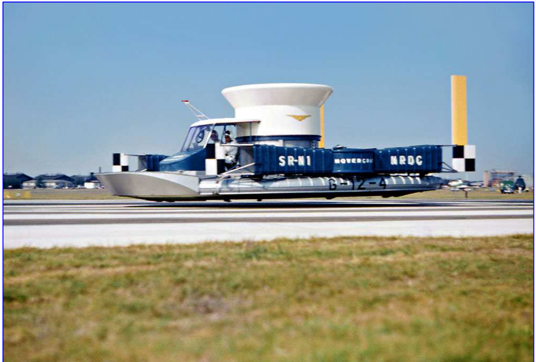
Figure 8.6: Modified Saunders-Roe Ltd SR.N1 Hovercraft (c) Exhibiting Daylight Clearance over Land
