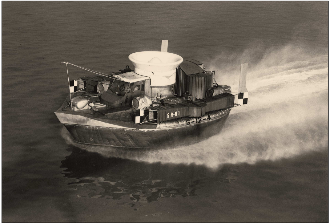
Figure 8.6: Modified Saunders-Roe Ltd SR.N1 Hovercraft (f) Fitted with 1.22 Meter Skirt
