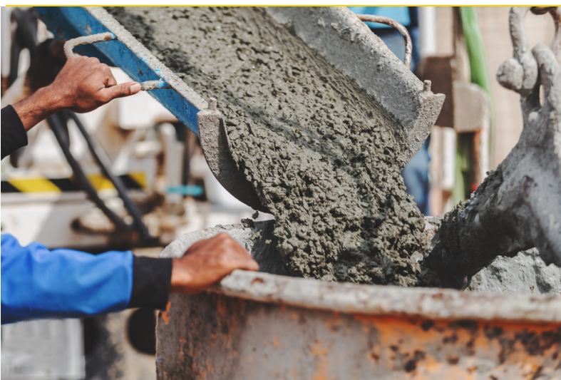
Photo is of concrete mixture being poured.
