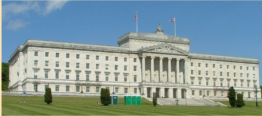
Photo: the Parliament Building at Stormont
