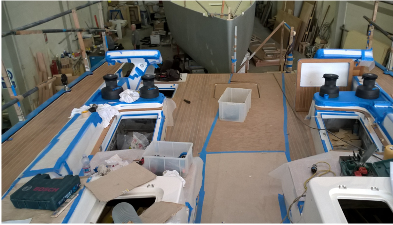
VISMARA-MILLS 62 deck equipment installation
