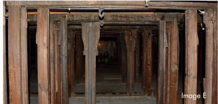
Image A: The lowest sub stage machinery with large drums and shafts. Image B: Fly loft with work bridges. Image C: Upper level fly loft. Image D: Winches below the stage. Image E: Chariots of the highest sub stage level.
