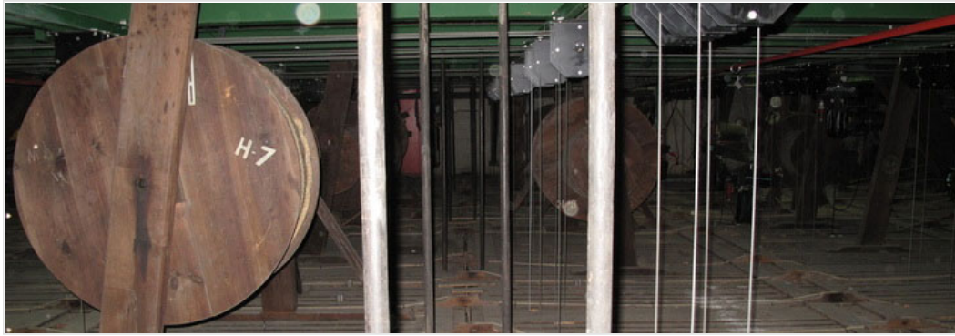
Historic and modern machinery side by side in the roof area above the stage
