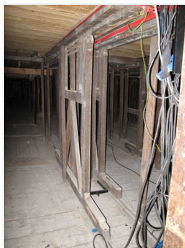
The level just below the stage is filled with chariots that once moved the wings on stage
