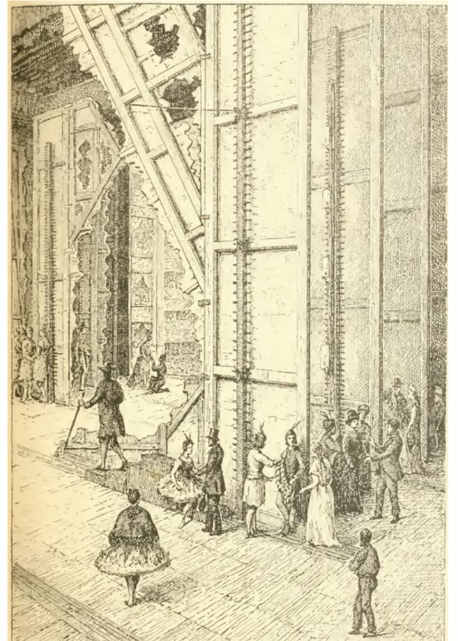
the movement, the next movement is prepared. The counter weights are pulled up by a winch, the control rope is pulled in again and the rope is changed to the other chariot. The set is now ready to move in the other direction.
