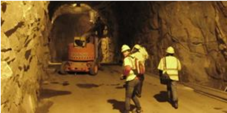
Figure 1: Inside one of the hydropower stations on the Lule River. Photo:M-B Öhmans
