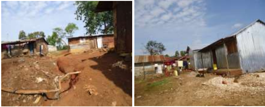
Figure 5: Examples of Houses in informal settlements
