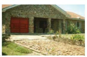
**Fig. 4:** An example of stone used as a maintenance free building material.
