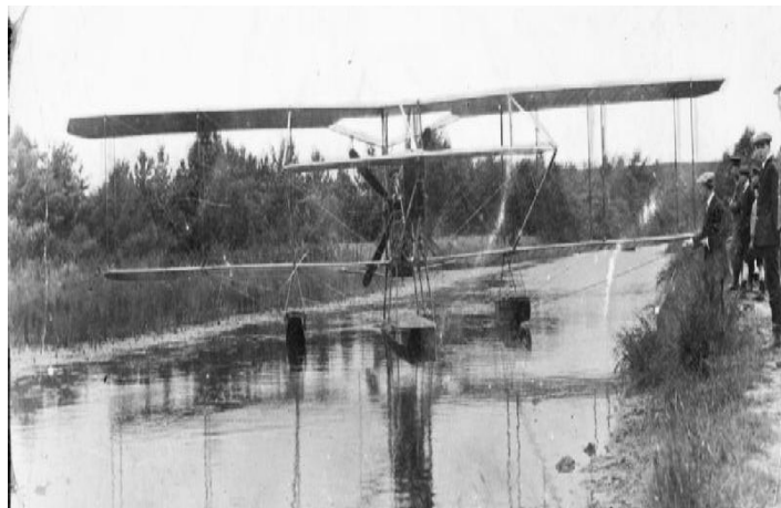
Cody aircraft mark VIB Hydroplane on the Basingstoke Canal, Cody at the controls. People on the tow path are pulling on a rope attached to the aircraft.
