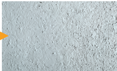
Base coat/crack-filling with KEIM Contact- Plus-Grob
