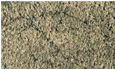
Existing render with cracks
