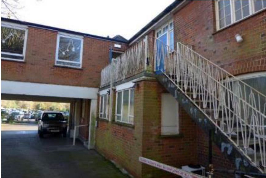
Fig. 41: View looking east, showing the external staircase, projecting toilet block and new assembly room added in 1967-8. (© Emily Cole)
