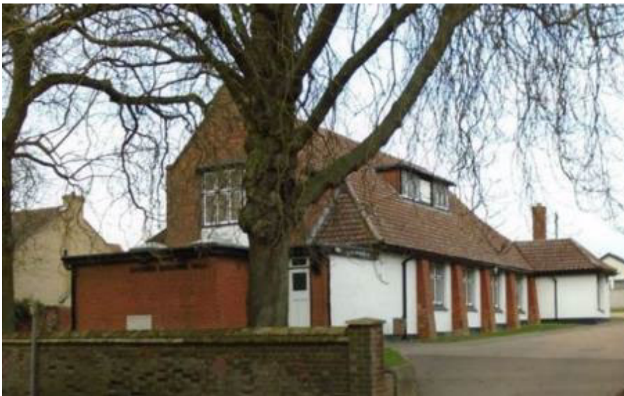
Fig. 68: The Gardiner Memorial Hall, Burwell, Cambridgeshire. Like the URC Hall, the building was designed by Spalding & Myers and completed in 1915. (Source: www.burwellparishcouncil.gov.uk/Gardiner_Memorial_Hall_-_Refurbishment_36616.aspx , acc. 12 Dec. '21)
