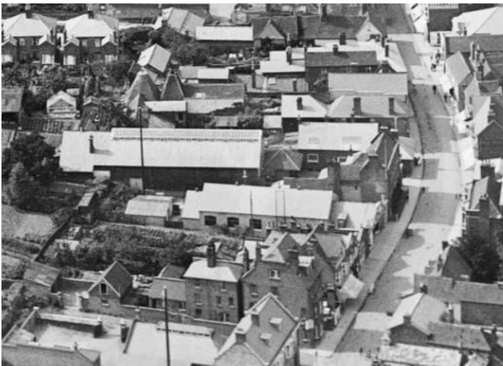
Fig. 22: Detail of 1920 aerial photograph, with South Street running south-north on the right. The Great Hall is at the centre left of the image, behind the working men's club. It was erected here in 1879 and demolished in 1937. (© Historic England, ref. EPW001740)
