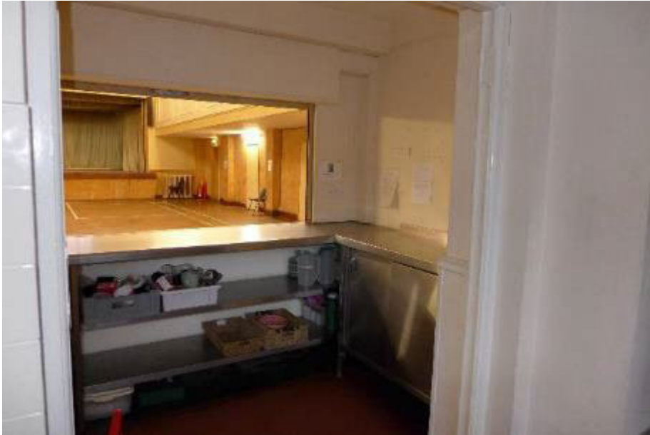
Fig. 52: Former doorway between the kitchen and the main hall, with double hinges visible on the right. The existing servery dates to the late 1960s. (© Emily Cole)
