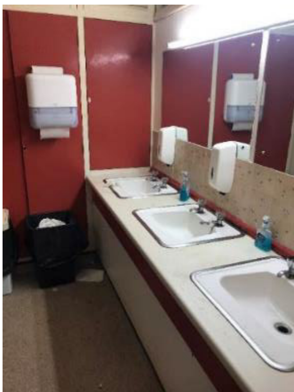
Fig. 48: The women's toilets as created in 1967-8, on the north side of the central hall. (© Emily Cole)
