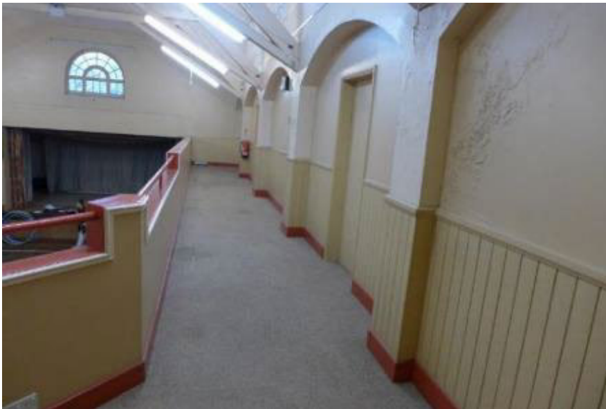
Fig. 51: View east along the south side of the gallery. Until the mid-1990s, the gallery contained tiered seating on two levels. (© Emily Cole)
