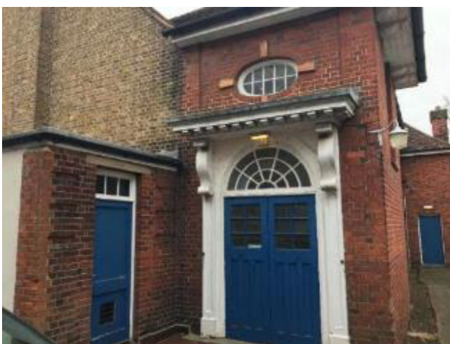
Fig. 33: The south-west entrance, with the projecting block containing the kitchen and boiler house on the left. The doorway on the far right provided external access to the large classroom in the south-east pavilion. (© Emily Cole)
