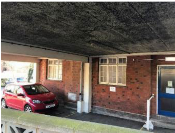
Fig. 42: The north side of the north-east pavilion as it appears today, after the remodelling of 1967-8. A foundation stone was reset in this area (left of central pier) and a new doorway inserted (right of photo). (© Emily Cole)
