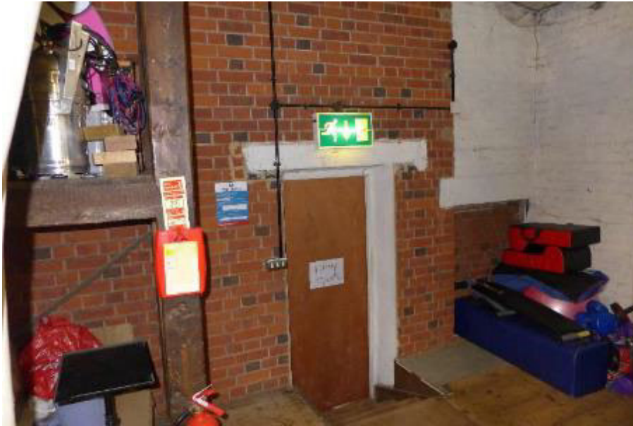
Fig. 28: The north side of the backstage area, showing one of the doorways created in the works of 1960/61. The brick wall was formerly external. (© Emily Cole)
