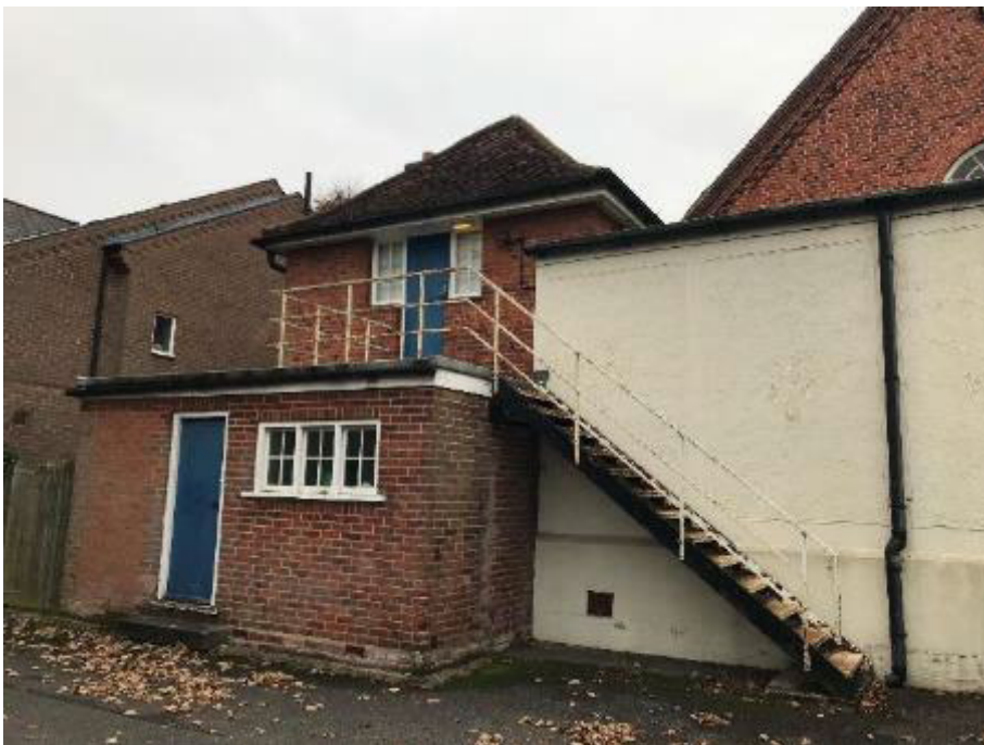
Fig. 25: View of the south-east pavilion of the URC Hall, with the expanded toilet accommodation and fire escape seemingly created in works of 1931/2. (© Emily Cole)
