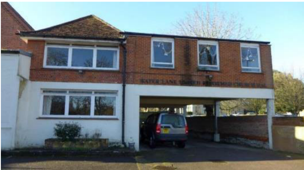
Fig. 38: The east elevation of the north-east pavilion (altered in 1967-8) and the projecting 'new room' (built in the 1960s phase of works). (© Emily Cole)
