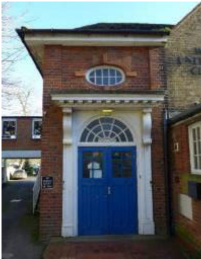
Fig. 32: The main (north-west) entrance doorcase and stair compartment, designed in the Neo-Georgian style. (© Emily Cole)
