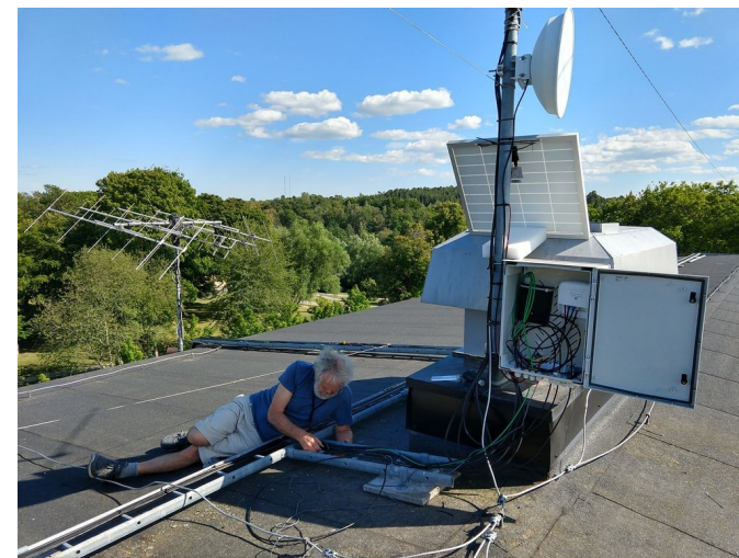
En typisk Amprnet-nod under installation
