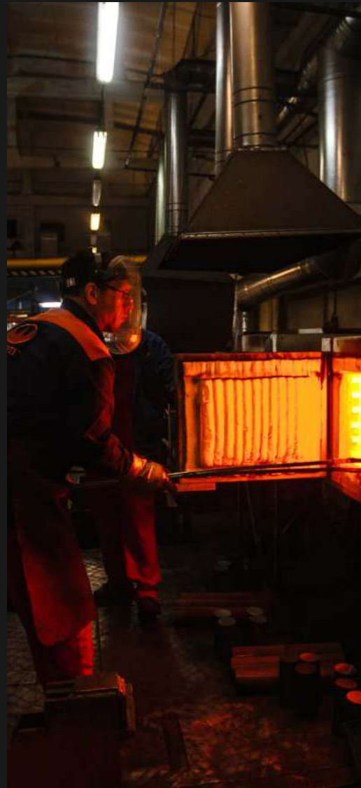
Welding on steel and aluminum, brazing of plastic structures, heat treatment.
