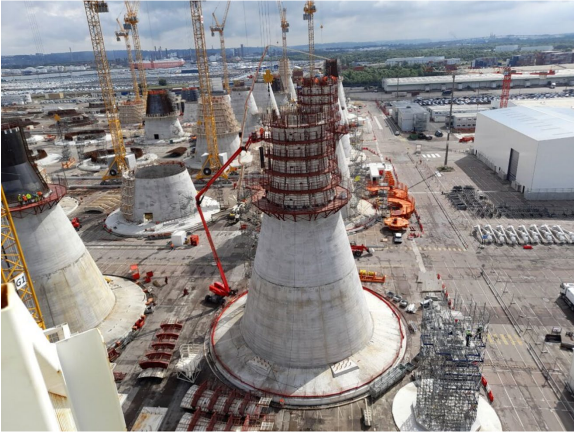
Figure I.3. GBFs under construction at the Fécamp project in France. 10
