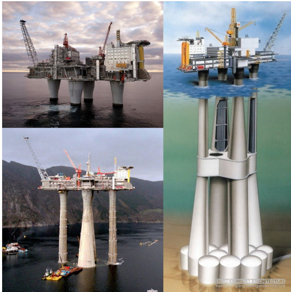
Figure I.4. The Troll A GBF platform was installed in 1996 and is operated by Equinor. With an overall height of 472 m and weighing 683,000 tonnes (1.2 million tonnes with ballast), it was the tallest structure ever moved by humankind. 13 (image credit 14 )
