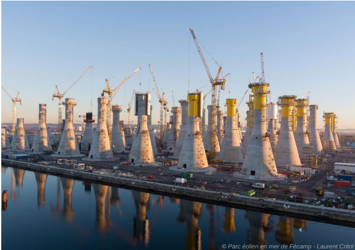
Figure 2.2: Concrete GBF Manufacture Site for Fécamp Wind Project in Le Havre, France. 66
