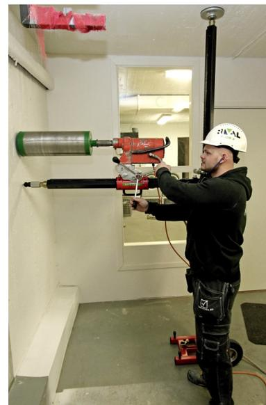
Horizontal drilling using 50<sup>+</sup> telescopic drill stand and Weka core drill motor.
