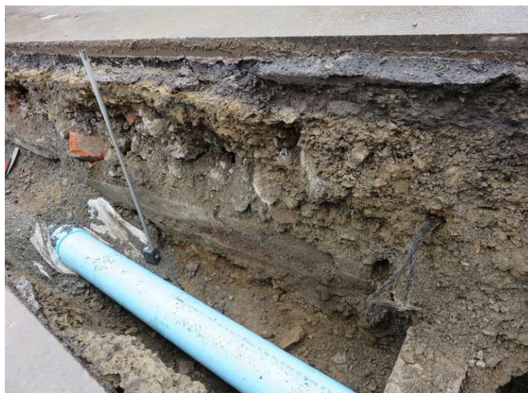
Illustration 32: Point P: concrete slabs (23 rd September 2015) (scale 500mm)
