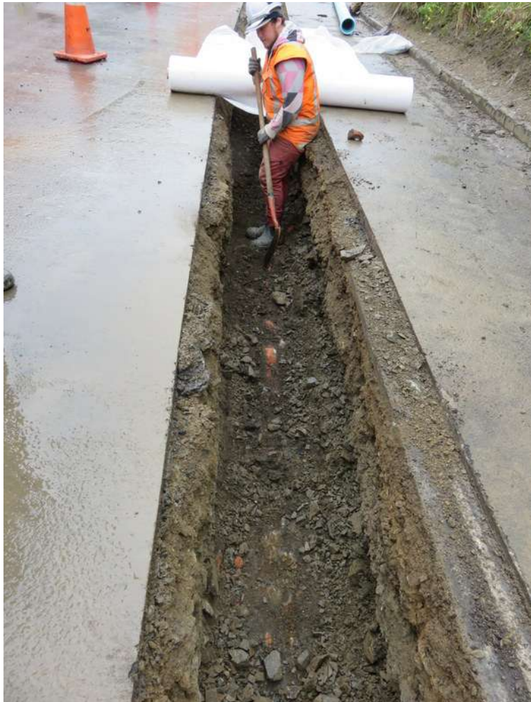
Illustration 35: North-east of Point Q showing darker fill material with bricks [L4] at base of trench (800-900mm) (23 rd September 2015) (scale 500mm)
