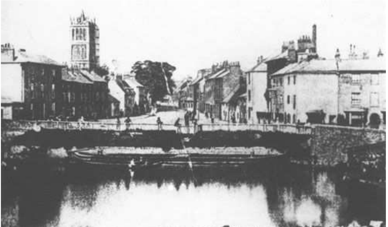
The former canal basin at Melton Mowbray. The entrance to the Oakham Canal can just be seen at the bridge on the right
