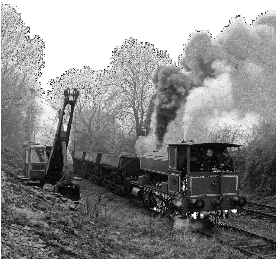
Left—1931 gets to grips with the dumper trucks as it shunts the quarry.
