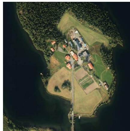
The main area of the prison is located in the centre of the island. Photo: Gule sider
