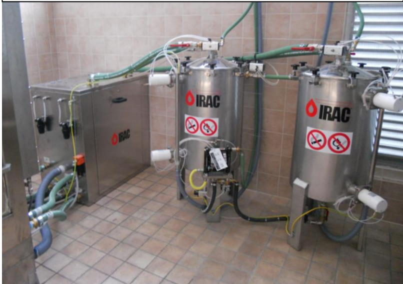
Pump box and feeding tanks with 150 lt. capacity each supplied with loading/unloading pump equipe with minimum and maximum level gauges interfaced with distillation plant mod. MAV 200
