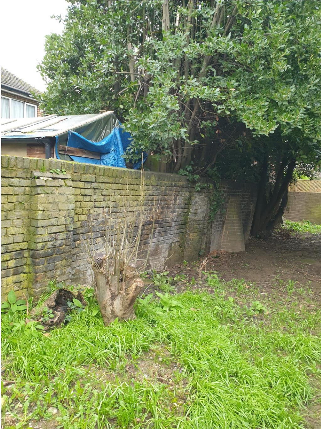
6.10 Group of trees on the other side of the wall, in the rear garden of a property in Presentation Mews. Note eroded pointing and remedial buttress.
