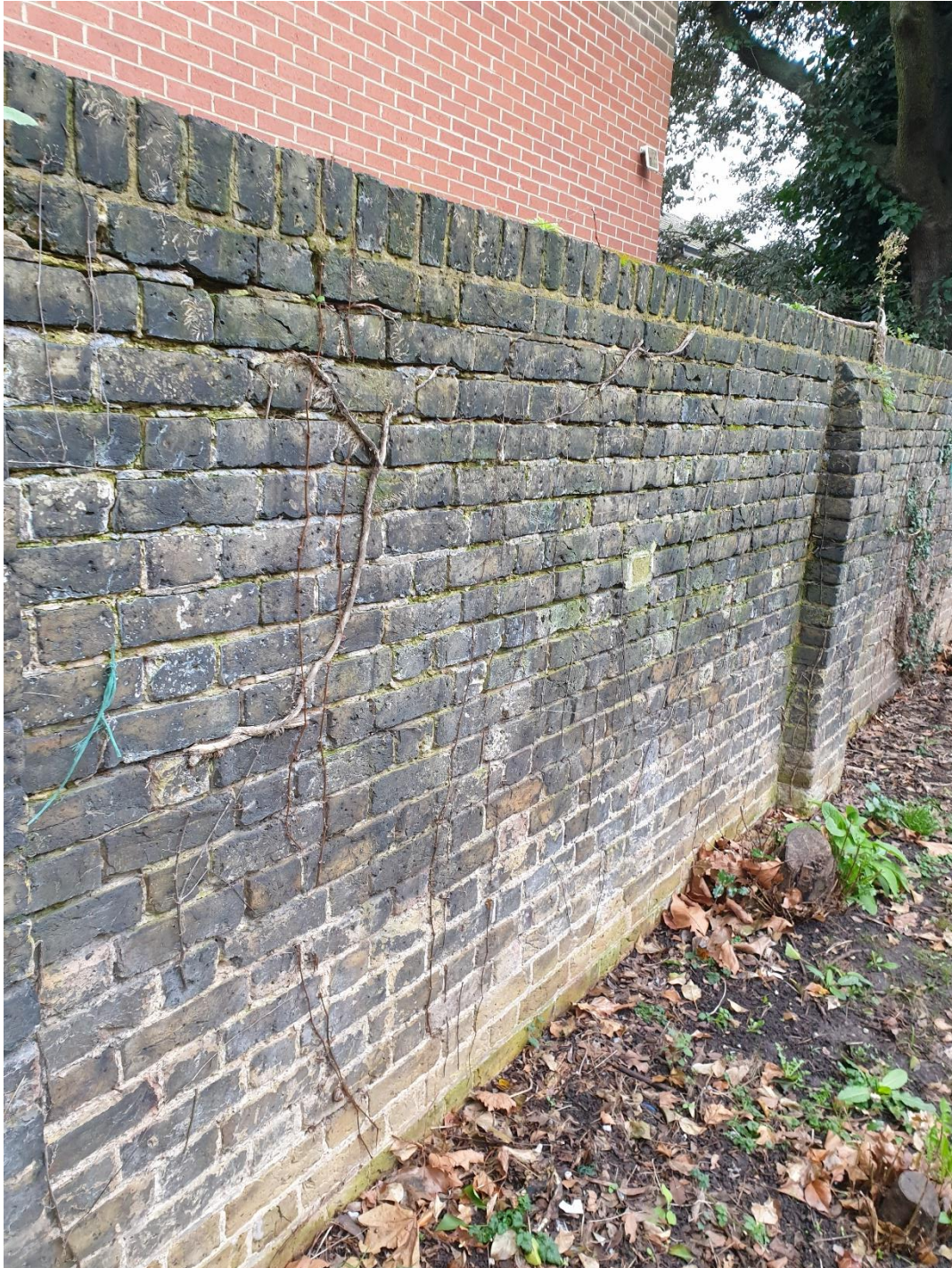
6.5 Eroded pointing and foliage growing out of the wall
