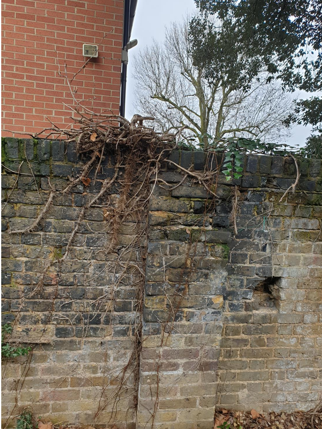
6.7 Eroded pointing, missing bricks and damage apparently caused by rootlets.
