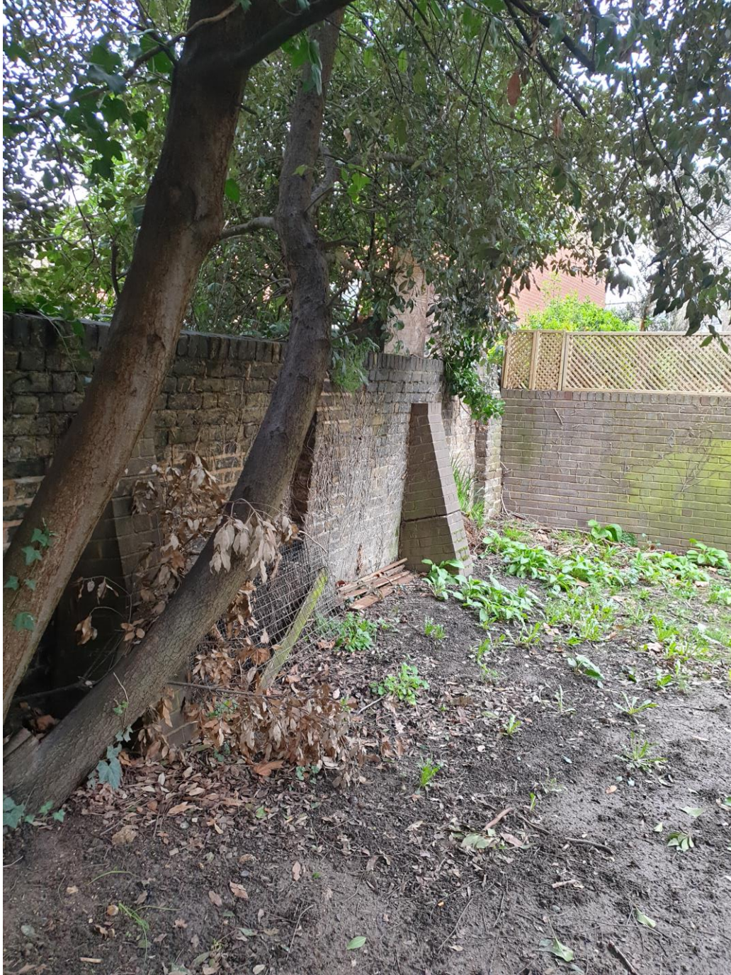
6.12 Fractured remedial buttress near north-east end of the wall.
