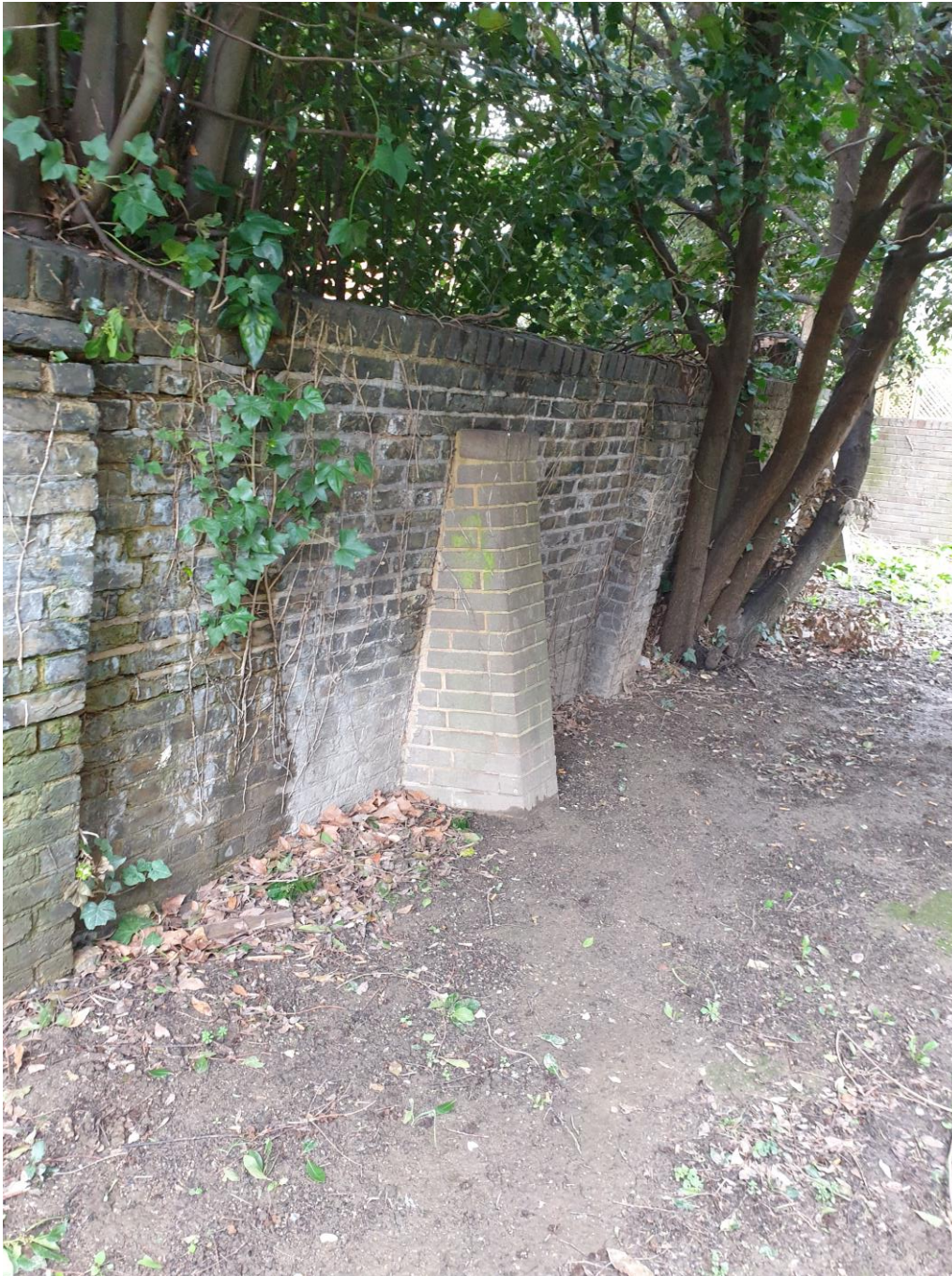
6.11 Remedial buttress. A second remedial buttress can be seen beyond the group of trees
