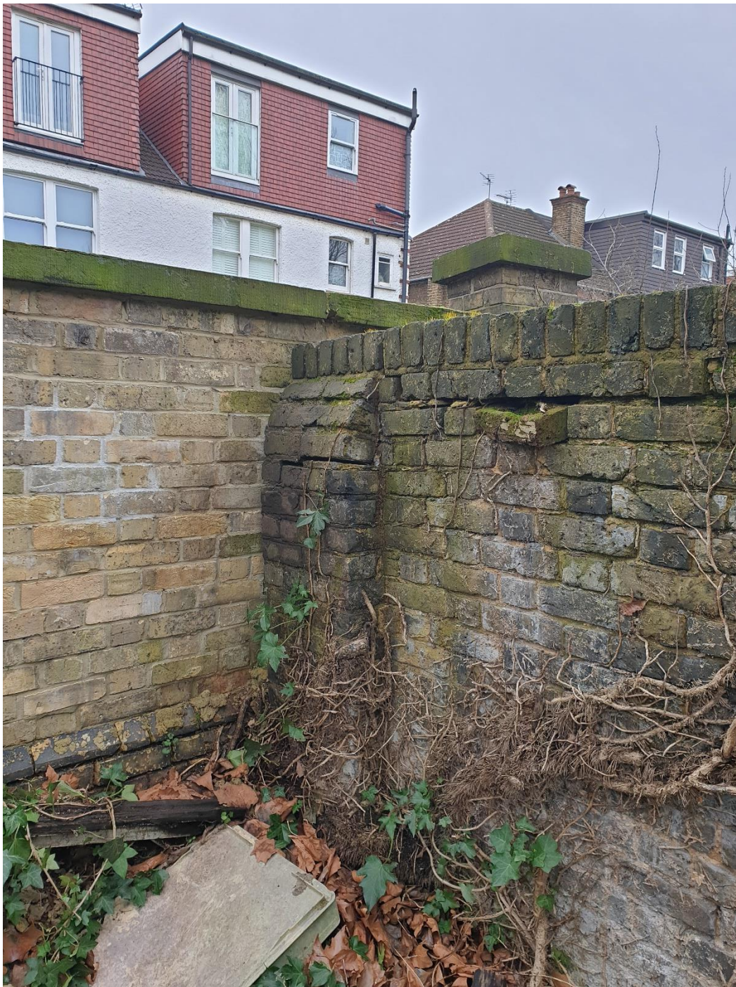
6.3 South-west end of wall. Note loose brick and eroded pointing
