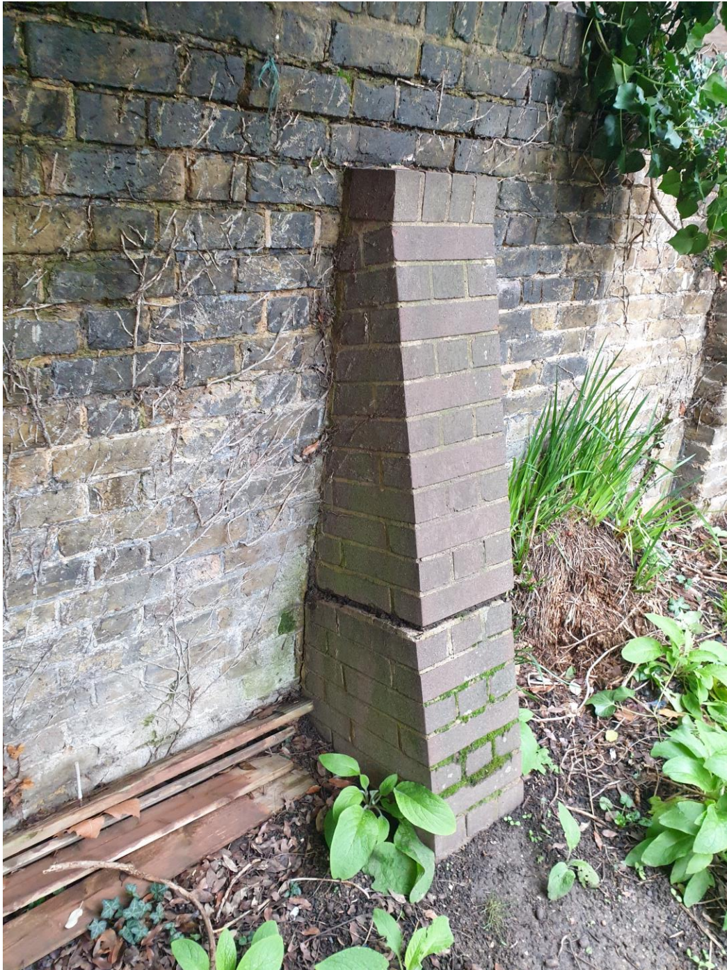
6.13 Fractured remedial buttress near north-east end of the wall.
