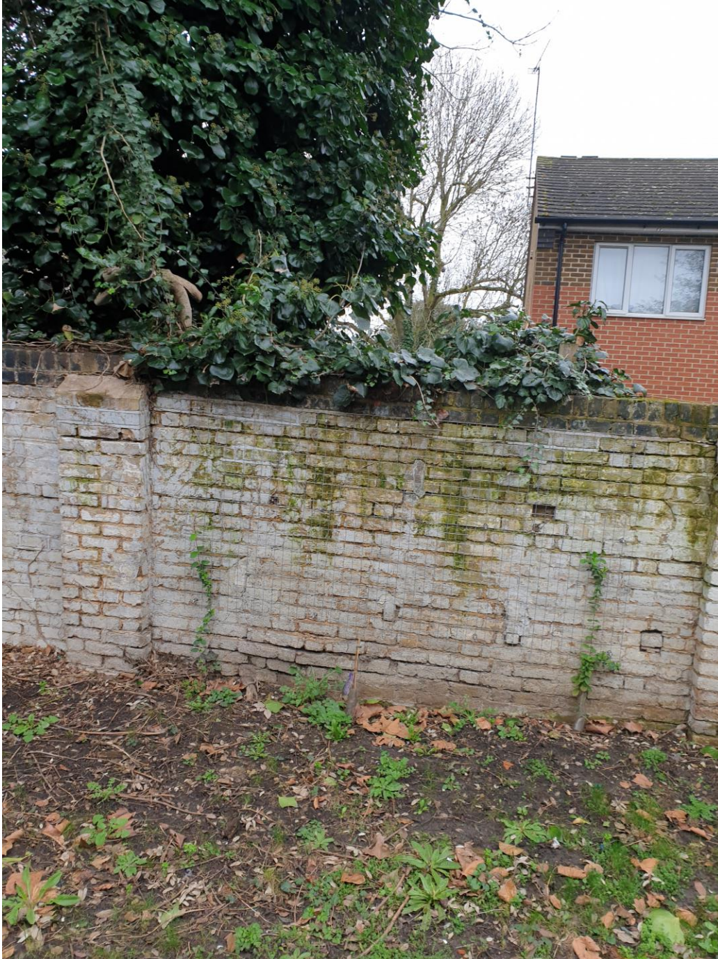
6.8 Eroded pointing.
