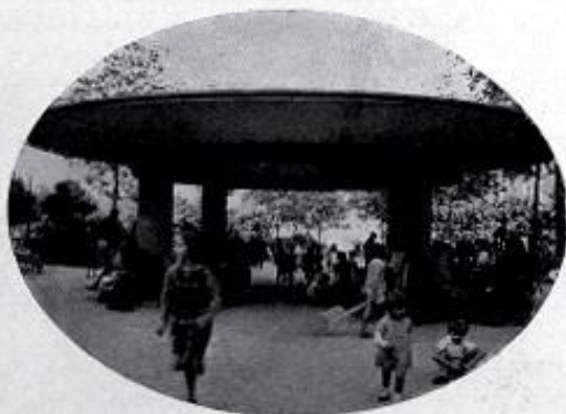
SQUARE SAINT-LAMBERT. ABRIS
