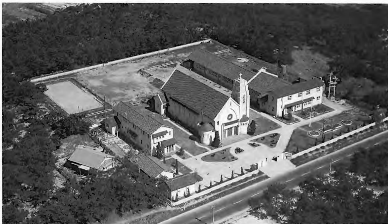
Koga Church, Rectory and Kindergarten
