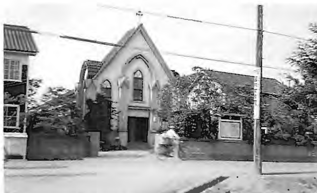
Enokuchi (Shinhonmachi) (original church)
