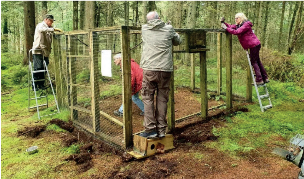
Figure 2. Volunteers building a release enclosure.
