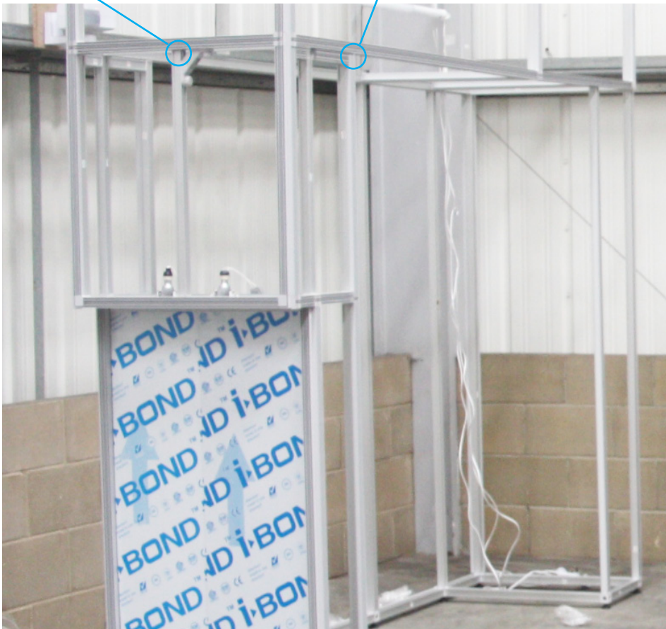
Vertical join to support a cantilevered lightbox.
