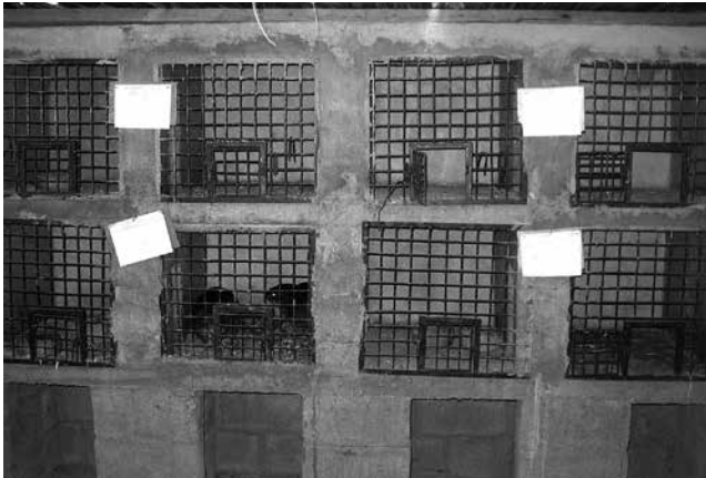
Figure 15: Two-layer concrete + cement-brick cages in a stable. Cages are constructed well above the floor to facilitate cleaning and tending. Cage height (above the floor?) is usually determined by the standard size of the cement-blocks; it could also be lower to allow three layers instead of two. Note marker tags on the cages.
