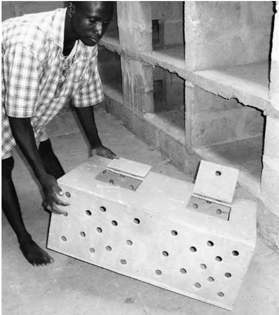
Figure 4: Grasscutter transport box in front of a concrete + cement-brick grasscutter cage under construction
