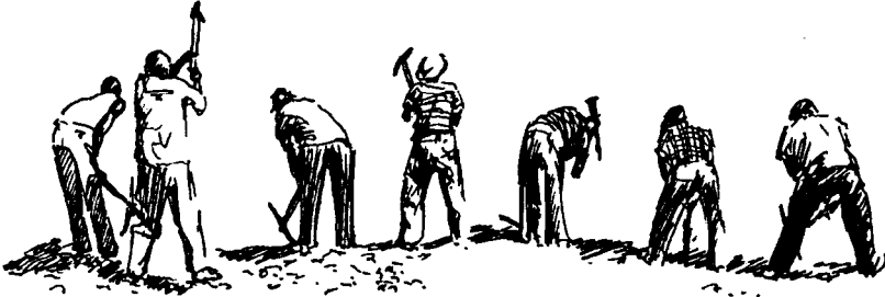
Figure 5: Digging a waterhole using labour-intensive methods.
