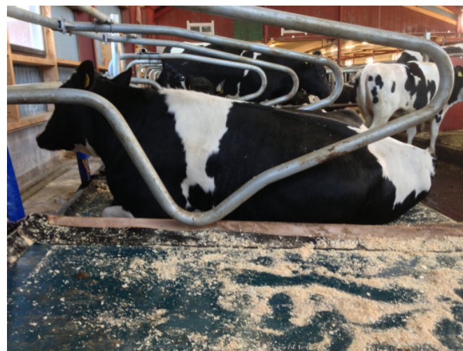
Cubicles installed in existing barn with scraper alley. Concrete edge 100 mm.
