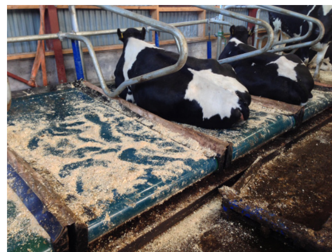
Cubicles installed in existing barn with scraper alley. Concrete edge 100 mm.
