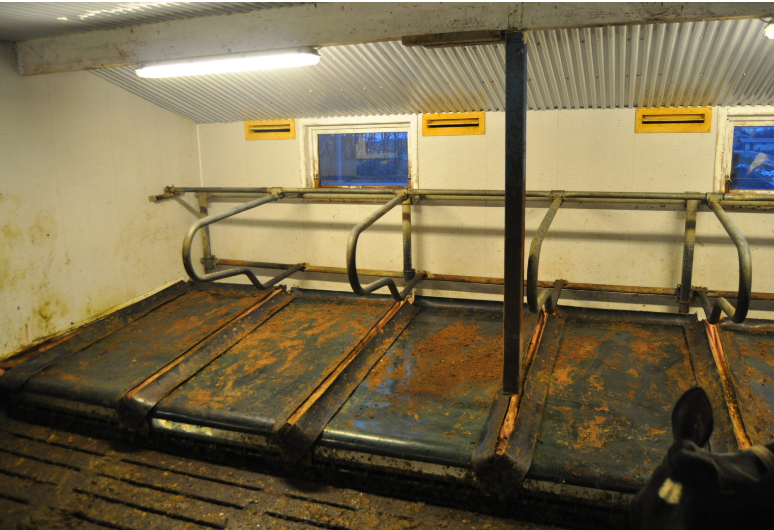
Cubicles with peat bedding. Installed with slatted flooring.
