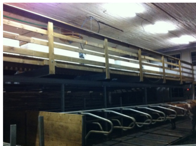
Groupboxes installed on a storey. Manure conveyor underneath the wooden walkway transports the manure out of the barn.
