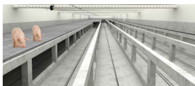
The conventional solution with slatted flooring means substantial ground and concrete works.
